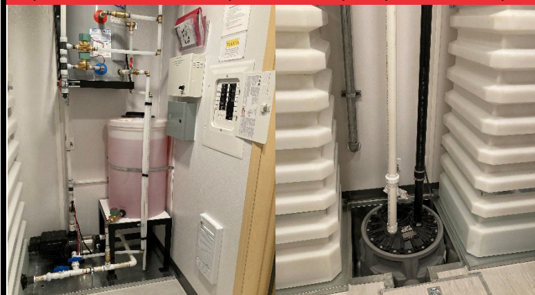
Glycol Freeze Protection System Heavy Duty Grinder Pump
